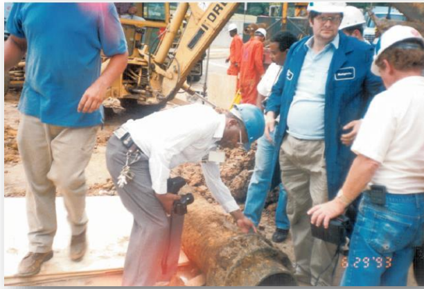
Cast iron replacement inspection
