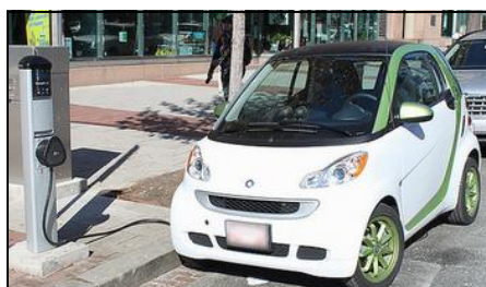
FC No. 1096– Electric vehicle charging at the Reeves Center.
