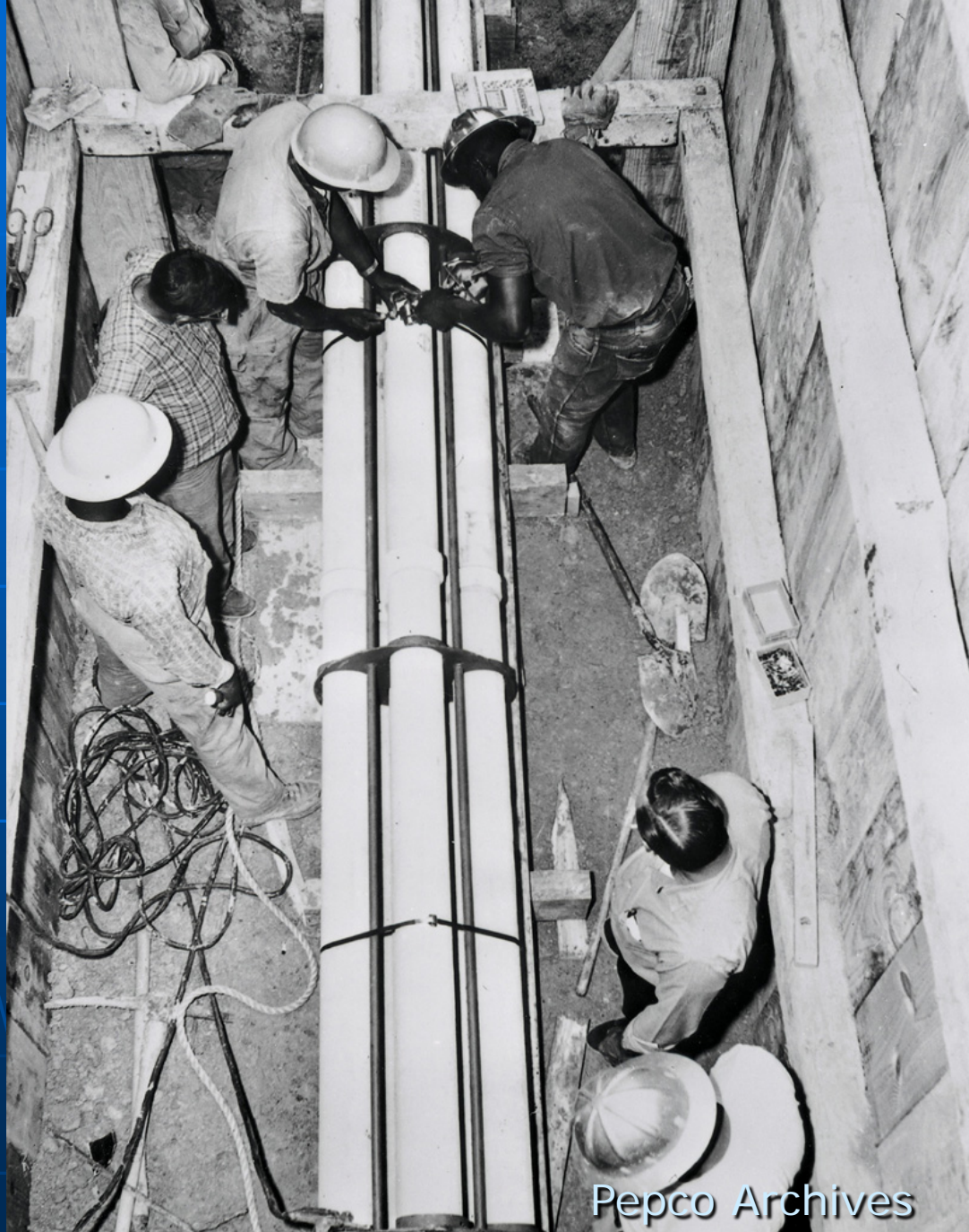
Installing new six-way conduit system, 1950s.
