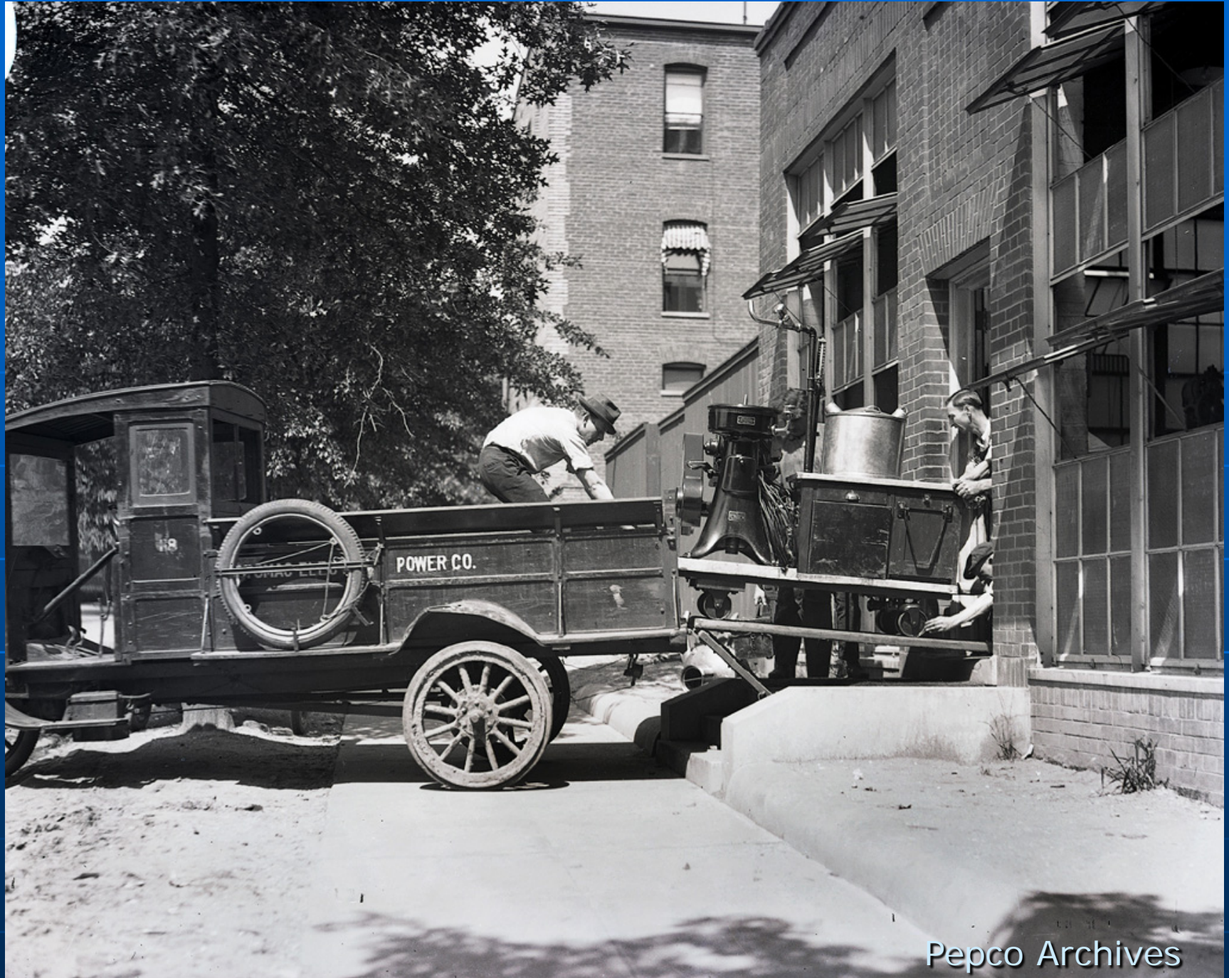
Unloading a direct current regulator into a substation ca. 1920.
