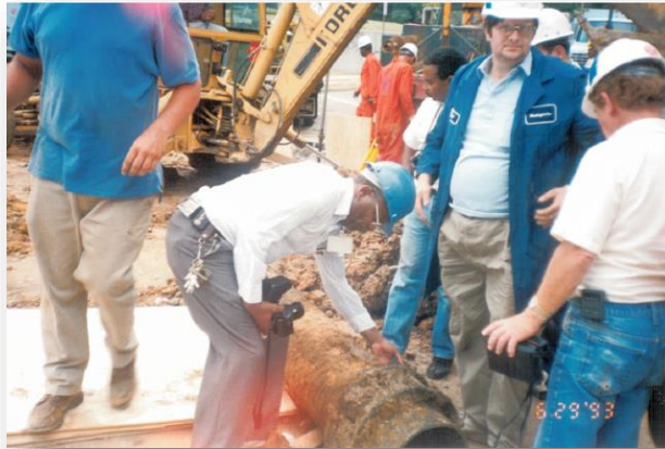
Cast iron replacement inspection
