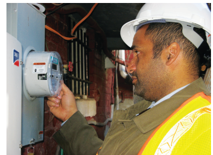
PSC Inspector Damon Patterson inspects a smart meter.
