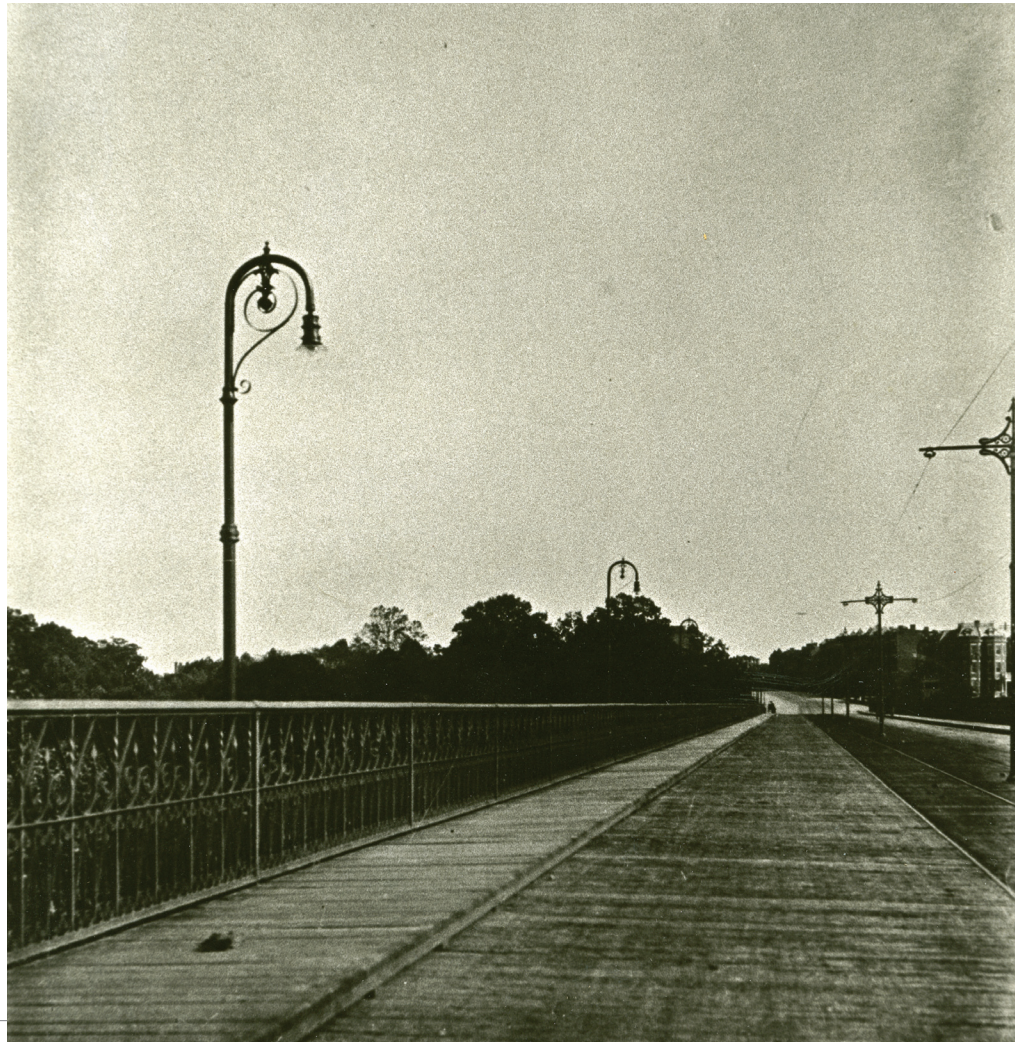
Calvert Street Bridge, lit by Pepco's "Newark Street-type" incandescent lamps, 1914.
