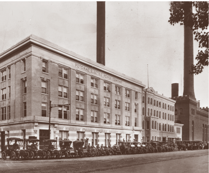
ABOVE: Potomac Electric Power Co.'s headquarters and power plant at Fourteenth Street and Constitution Avenue.
