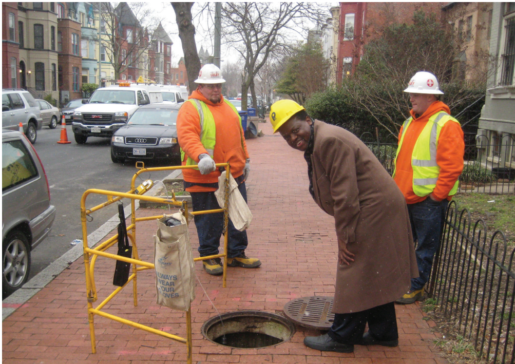
PSC Chief Engineer Udeozo Ogbue inspects a manhole.
