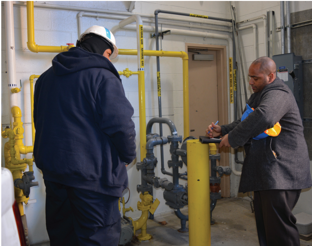
PSC Inspector Damon Patterson conducts a natural gas inspection.
