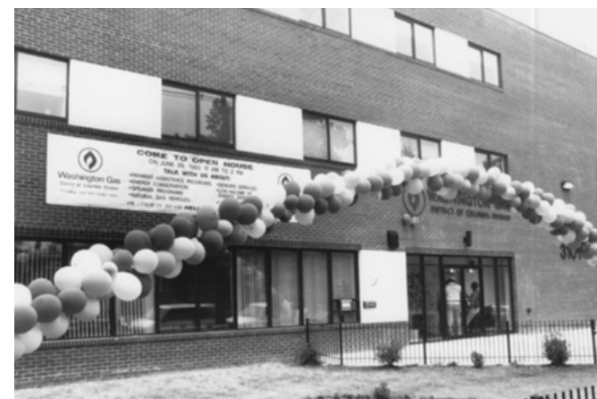
WGL's Customer Service Center in Ward 8
