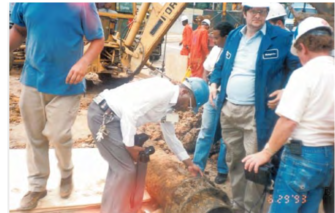
Cast iron replacement inspection
