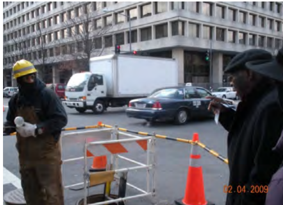
Dr. Joseph Nwude, deputy executive director for regulatory analysis (at right), conducting a manhole inspection.
