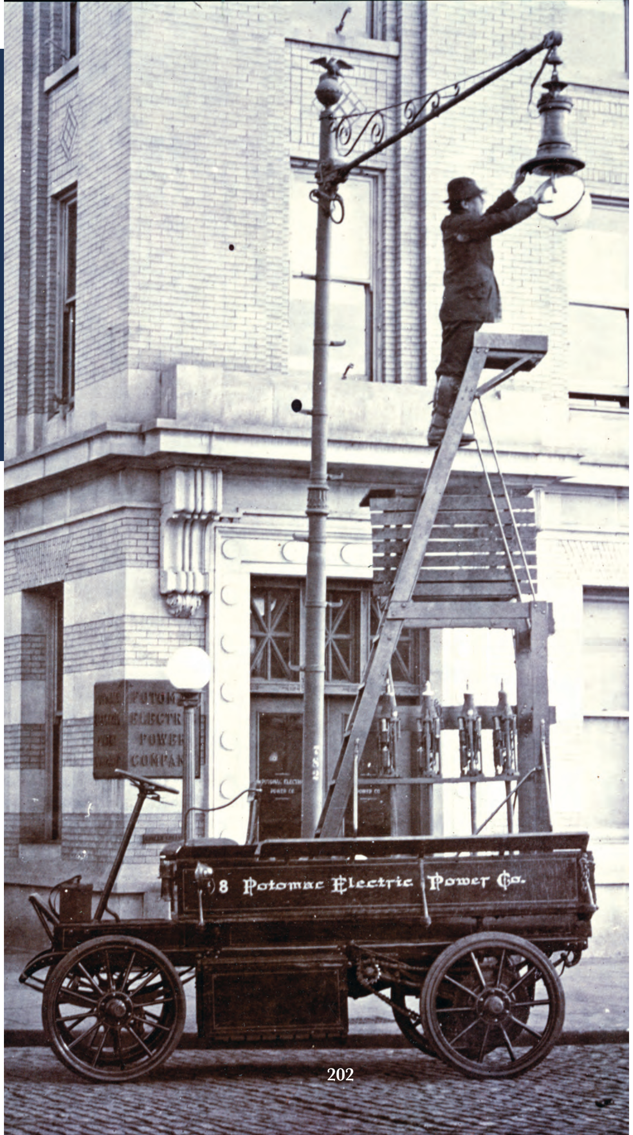
A Potomac Electric Power Co. employee uses a scaffold mounted to a service truck to change an electric arc streetlamp in front of PEPCO headquarters at Fourteenth and B (Constitution Avenue) streets, about 1915. Historical Society of Washington, DC
