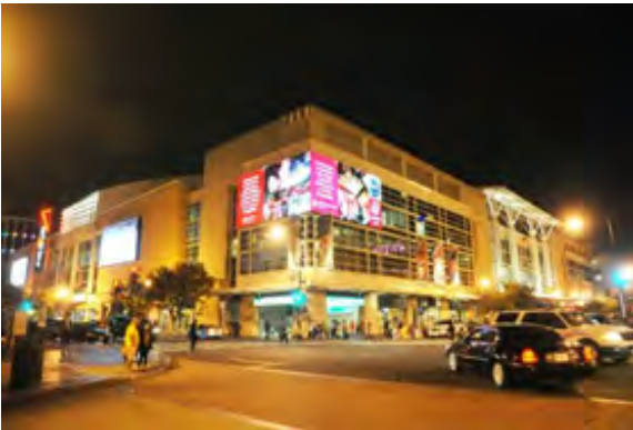
Verizon Center, Northwest
