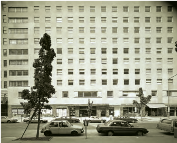
Cafritz Building, 1625 I Street, Northwest, 1963–1980
