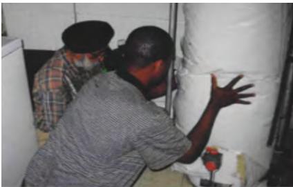
PSC staff, Manmohan Singh and Damon Patterson, insulating a consumer's water heater.
