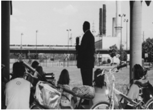
River Terrace activist, George Gurley, led opposition to PEPCO adding generators to its Benning Road plant, 1987.
