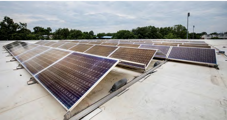
ROOFTOP SOLAR PANELS ON FRANK W. BALLOU HIGH SCHOOL (WARD 8)
