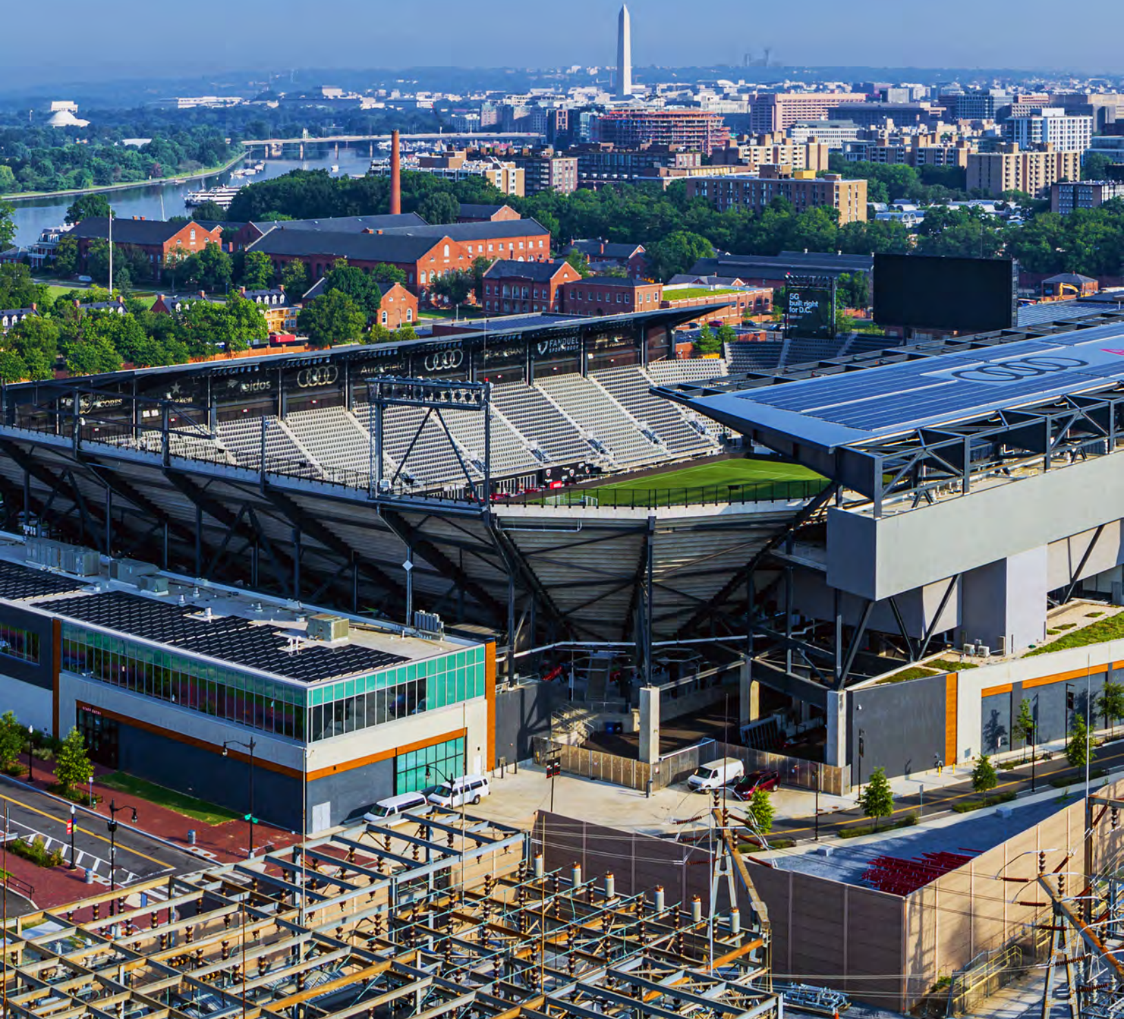
Audi Field rooftop solar installation and Pepco Buzzard Point Substation (Ward 6)
